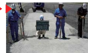
出来形検尺 Measurement of the completed part 检查完工尺寸
